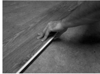
Fig. 4 – Angle long side into prior row.
