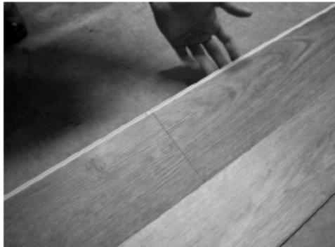
**Fig. 6 - Locking long side with ends already locked**
