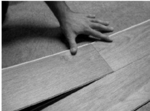
**Fig. 5 - Angle end of next plank**
