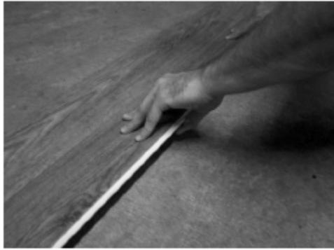
**Fig. 4 - Angle long side into prior row.**
