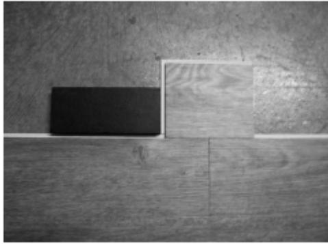
**Fig. 7 - Tap side of plank with tapping block**
