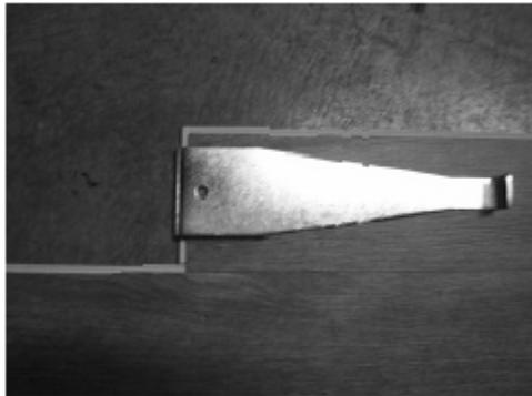
**Fig. 8 - Tap end of plank with pull bar or tapping block**
